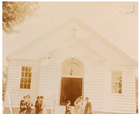
Messiah, Decatur, 1st Building 1936
