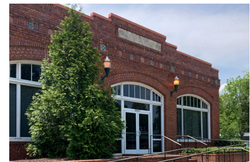
Survey Publishing Company Building
